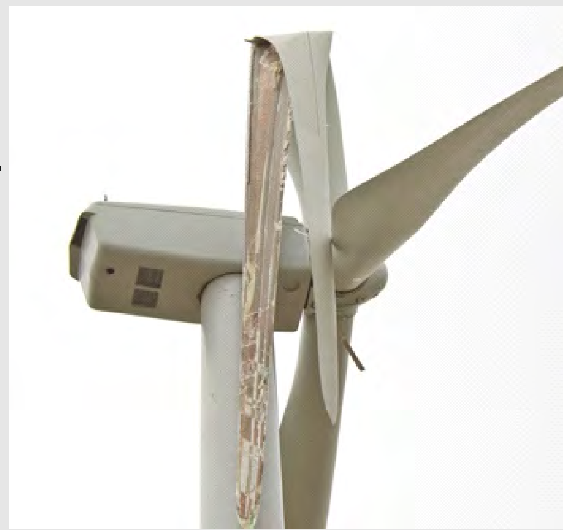
Defektes Rotorblatt (Totalausfall) http://basinelectric.wordpress.com
